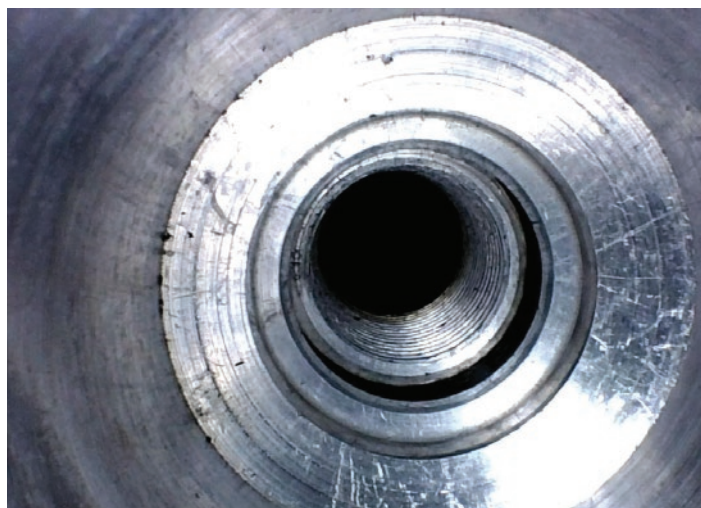
Photo above: Spark plug port inspection
