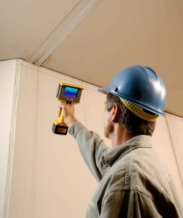
A technician checks the extent of moisture damage.
