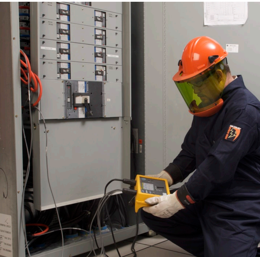
Testing power on a distribution panel.
